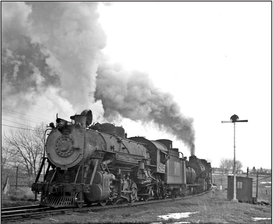
Denver & Salt Lake 405, along with a big D&SL articulated, stop at the west siding switch of Leyden to receive orders on their way down the hill into Denver. – Photo from the Nathan Holmes collection.
